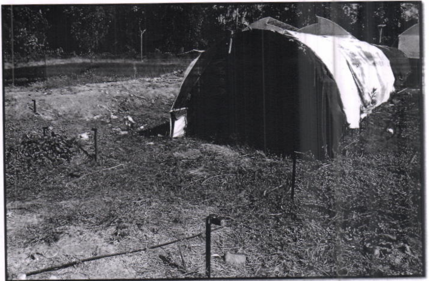
Tunnel Shed No. 2
